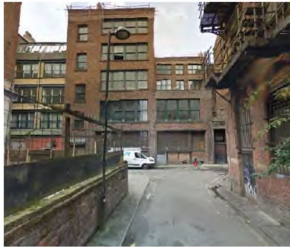
existing view from mangle street to back piccadilly
