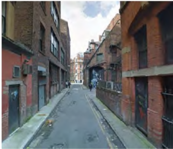
existing view from back piccadilly to newton street
